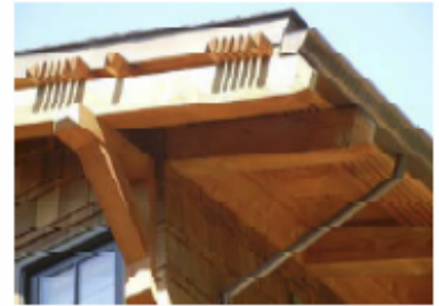
Building with copper flashing, gutter and drainpipe.
