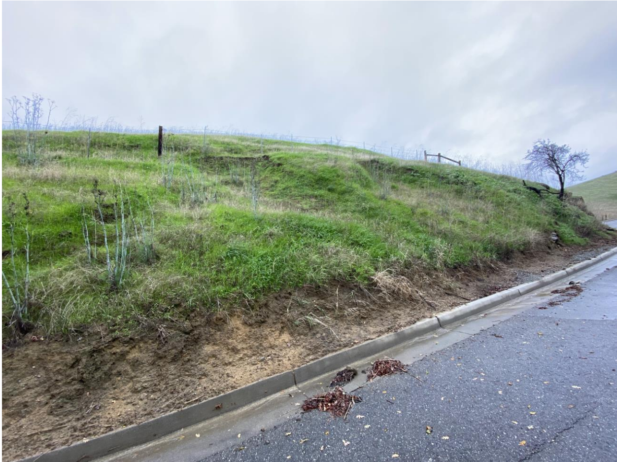
Shallow landslides along slope adjacent to paved access road to Solano Irrigation District Water Reservoir
