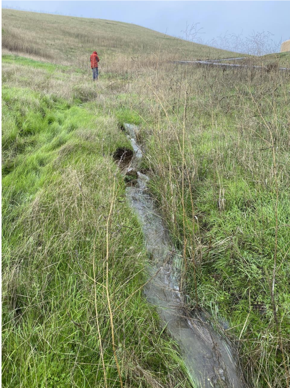
Erosion gully south of access road to Solano Irrigation District Water Reservoir
