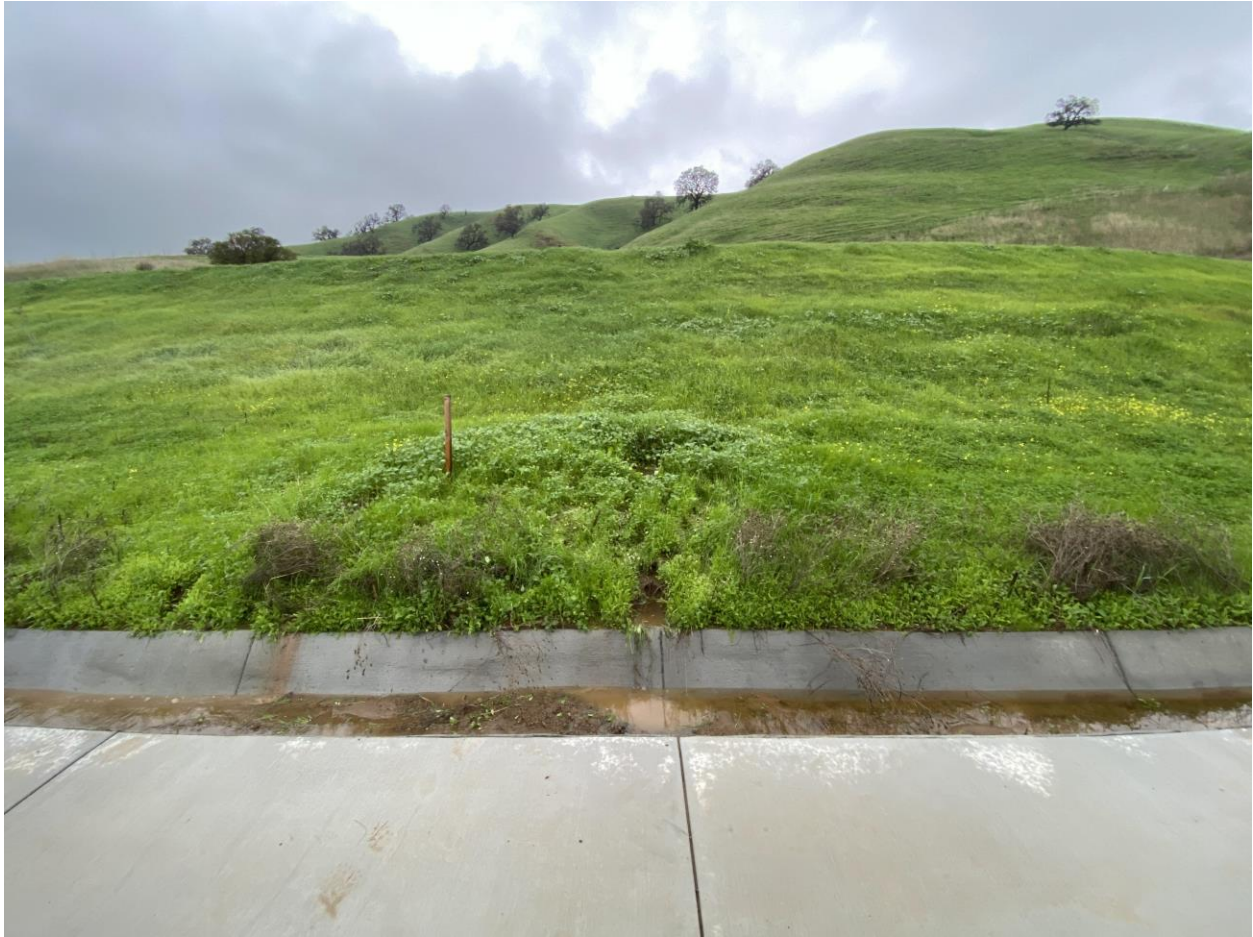
Buried pipe outlet apron from Sedimentation Basin "I"
